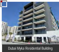
Dubai Myka Residential Building
